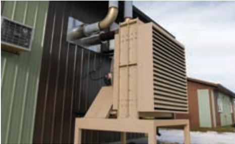
The 750 kW generator from MTU Onsite Energy is installed in the equipment room along with the switchgear, while the radiator is installed outside to reduce heat buildup.
