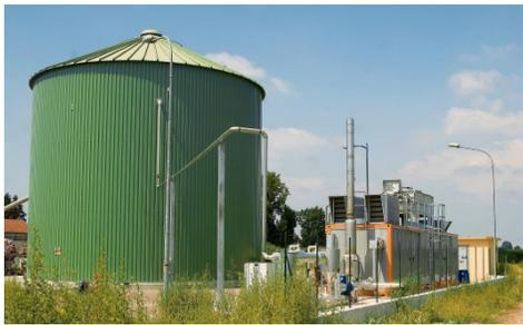
Corn and liquid manure ferment in a tank to produce biogas which powers the CHP plant.
