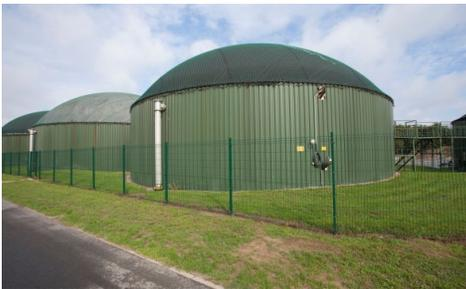
The company GF-Bio-Energie Hasetal GmbH in Lönningen. 60 tonnes of renewable energy crops, 60 tonnes of slurry and 10 tonnes of manure are fermented every day in the biogas plant.
