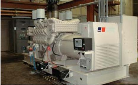
MTU Onsite Energy standby power systems installed at Fairfax County wastewater pumping stations operate at 1,800 rpm, or twice the speed of the units they replaced. The new generators also feature state-of-the-art electronics and will start and accept load within 10 seconds.
