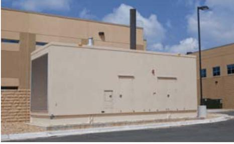
The power system consists of an MTU Onsite Energy 2000 RXC6 DT2 Series 4000 generator set, a digital master control, automatic transfer switches and associated switchgear. The standby generator itself is located outside in a sound-attenuated enclosure that was necessary because the enclosure is located adjacent to a part of the building that houses the judges' chambers.
