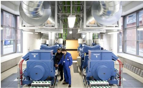
The two generator units are based on MTU type 12V 4000 G23 diesel engines with a combined electrical output of roughly 1,700 kVA and can be up and running inside ten seconds.
