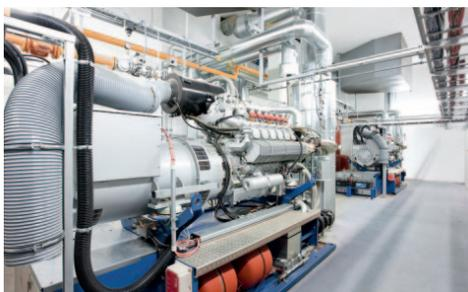
The two type GC 357 N5 CHP plants equipped with MTU Series 400 engines deliver around one megawatt of thermal and approx. 700 kilowatts of electrical energy.
