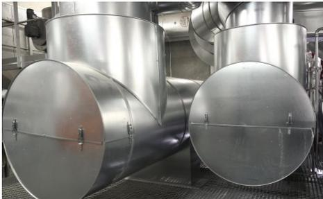
The low-temperature exhaust gas heat exchanger (right) boosts fuel efficiency by an additional three percent.
