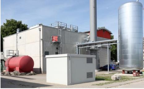
In order to handle the cogeneration module's higher electrical power, a 0.4/20kV transformer (seen in front) was set up in the combined heat and power station.
