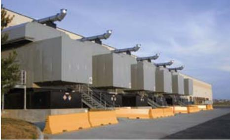
Critical data centers consume prodigious amounts of electric power to run servers and the air conditioning needed to get rid of heat the servers produce. This means backup power systems must be designed to handle considerable loads.
