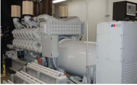
Two MTU Onsite Energy 2,250 kW generator sets back up the main data center for Synovus Financial. The generator sets can start and assume full load in under eight seconds thanks to about 20 percent more cylinder displacement per unit of horsepower than other generator drive engines.
