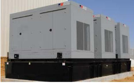
All three generators sit on top of a single 7,500-gallon fuel tank that provides a 72-hour runtime and reduces hassles during refueling.
